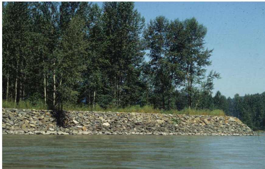
Figure 10. Well-constructed rip-rap placed to prevent bank erosion. This rip-rap protects a hydroelectric power line pylon.
