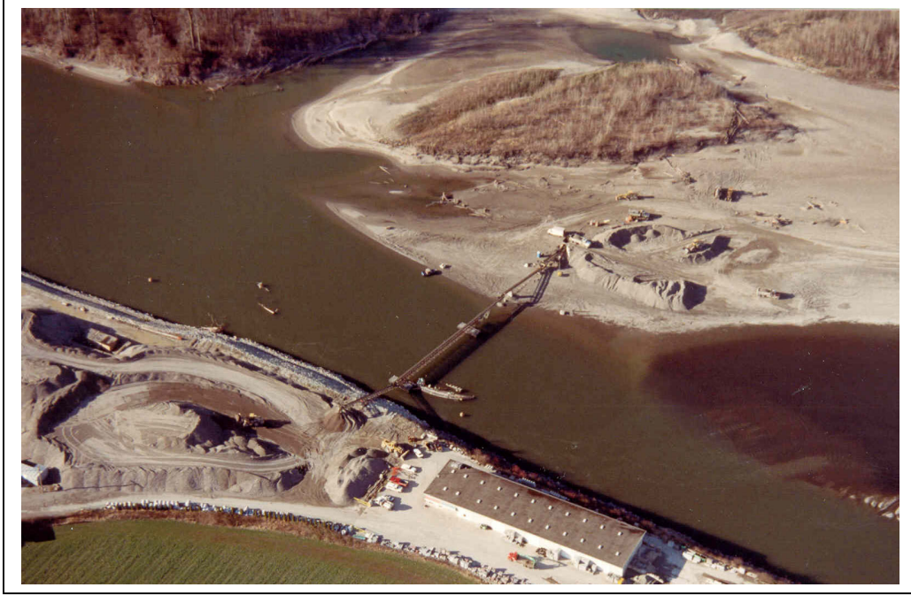
Stockpile area and conveyor belt used to transport gravel from Minto Island to Steelhead Aggregates Ltd. yard. Photograph taken March 6, 2000 (courtesy of Dr. V. Galay).
