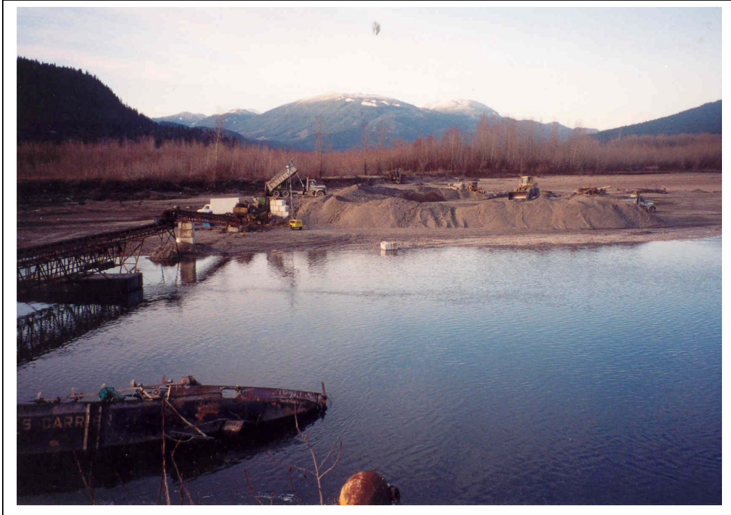
Gravel stockpile and conveyor belt across Minto Channel (March 7, 2000).
