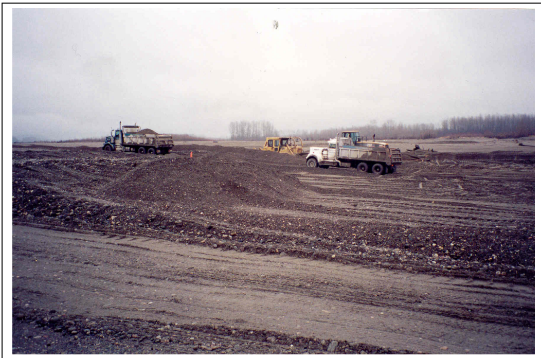
Ground view of scalping operation at Harrison Bar. Photograph taken March 7, 2000.
