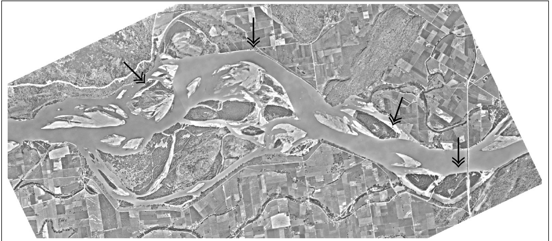
Figure 4 Island 32 and vicinity, May 7, 1962; Hope flow 2,940 m 3 /s. Source Resource Surveys and Mapping Branch, British Columbia Ministry of Environment, Lands and Parks. Arrows indicate sites of erosional attack.
