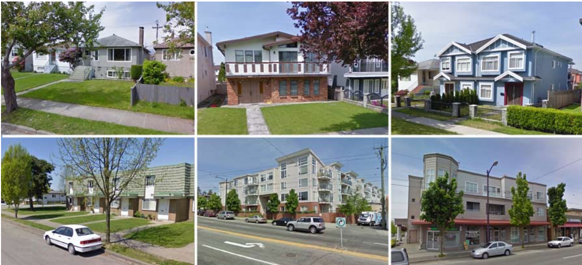
Figure 2.1.2: Illustrative photos of principal dwelling types within study area. Clockwise from upper left: pre-1965 single family bungalow; 1965 – 1990 single family with secondary suite option; duplex; rowhouse; apartment; and, mixed use. Images generated using Google Maps and Streetview ( http://maps.google.com/ ).
