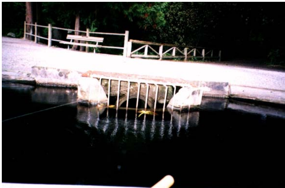
Figure 5-8 Main weir on Beaver Lake
